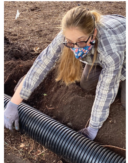
Sarah Zipfel adjusting the slope of the drain pipe
