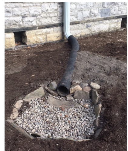
-Completed downspout water area
