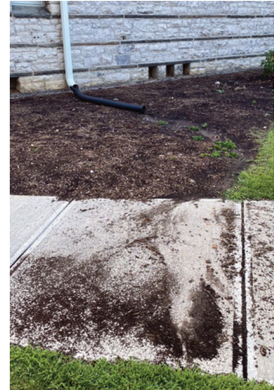
Soil washing off of the site when there is a hard rain
