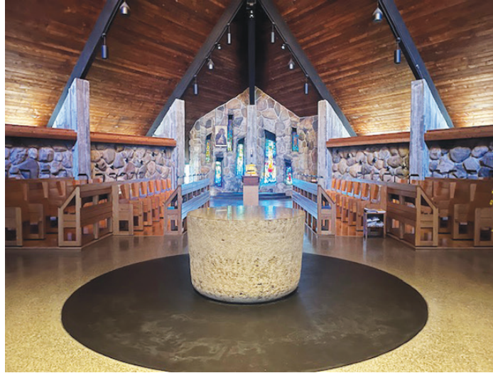
The chapel at the Abby of the Genesee constructed with stones from the neighboring farmlands which were prepared by an acid wash.
